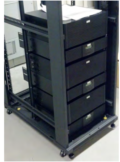
Figure 2. Supercapacitor system modules are designed to easily fit into standard 19" racks. The modules can be stacked as well.
